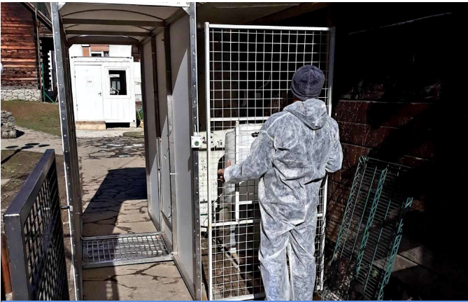
Disinfection tunnel in TRC Sedra isolation area © IOM 2021
