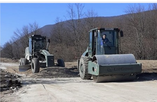
Works on access road to Lipa © BiH Army 2021
