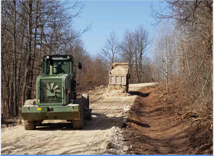
Works on access road to Provisional Camp Lipa © IOM 2021
