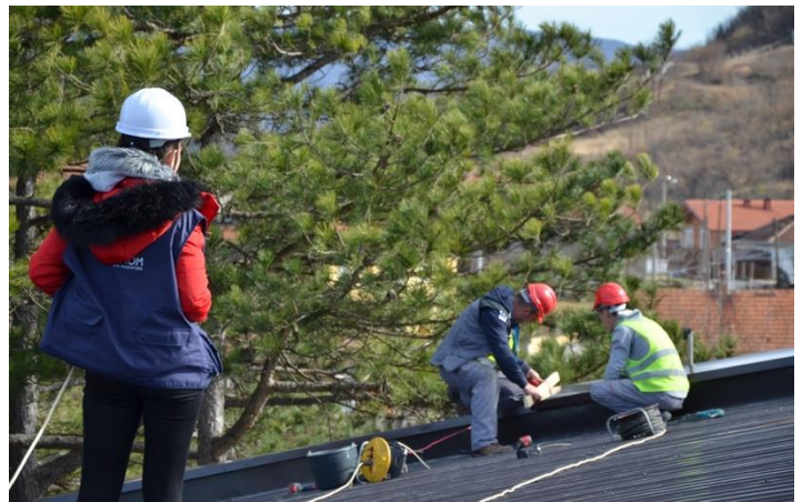
Repairing the roof in TRC Borici, IOM
