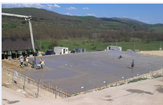
Works on the dining area in TRC Lipa © MoS, IOM 2021
