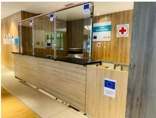
Renovated dining hall in TRC Sedra © IOM 2021
