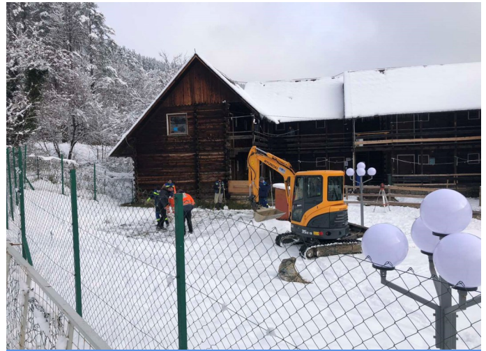
New sanitary containers installation in TRC Sedra © IOM 2021
